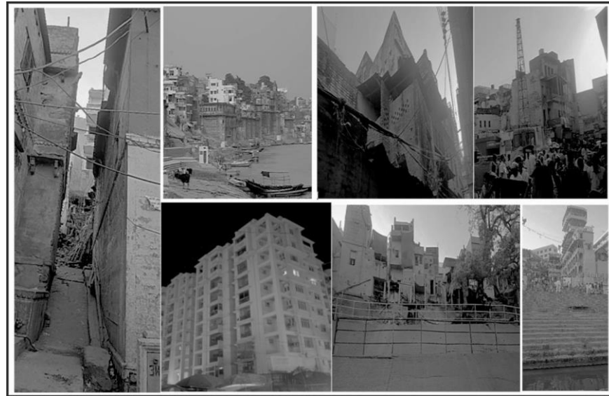
Figure 3. Building typology of the Varanasi city (Uttar Pradesh, India)
