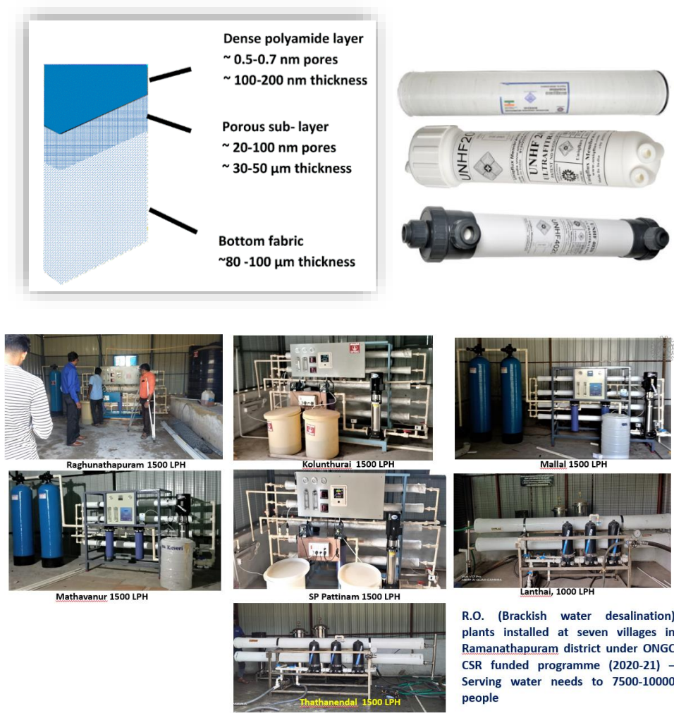
Figure 4. TFC membrane, module and recently installed few RO desalination plants as per CSIR-CSMCRI membrane design (2020-2021).
