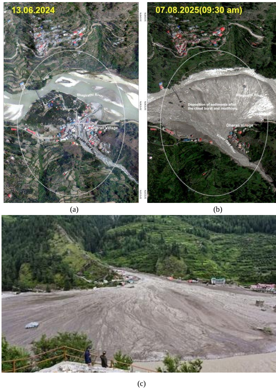
Figure 4. Satellite images of Dharali village showing picture of (a) before, (b) after flash flood, released by Indian Space Research Organization (ISRO). Dharali settlement occupies portions of an alluvial-fan/floodplain surface and (c) The Dharali town which was completely washed away after flash flood and alluvial fan of Khir Gad. This photo shows Kheer Ganga where formation of alluvial fan took place after dumping the huge amount of debris load that reshaped its old channel/alluvial fan during flash flood
